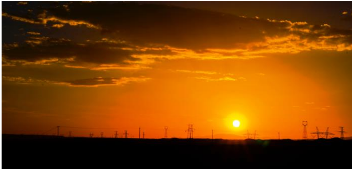
Qing Yu UHV DC spans up to 1563 km, enabling sunlight from the northwest plateau to light up households in the central plains.
