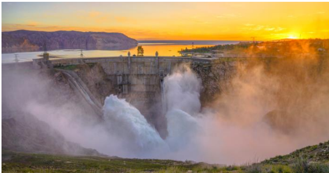
The first major power station on the Yellow River – Longyangxia Hydropower Station
